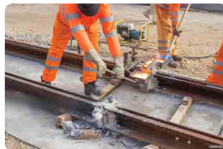
Figure (7) Welding rails using the thermite reaction.
